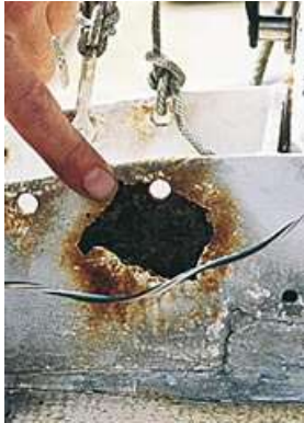
Figure 3. A large rust patch was started by water getting under the protective paint work at the edge of the hole and has resulted in substantial damage.
